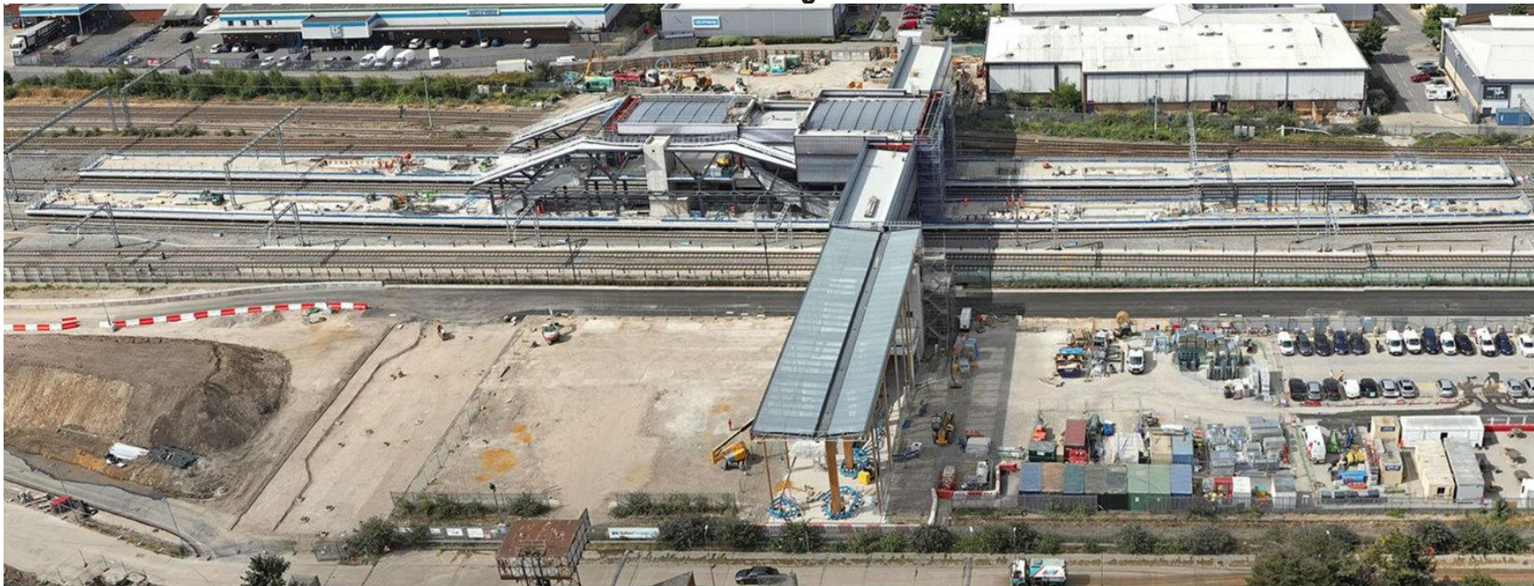
BXW Station looking East to West
