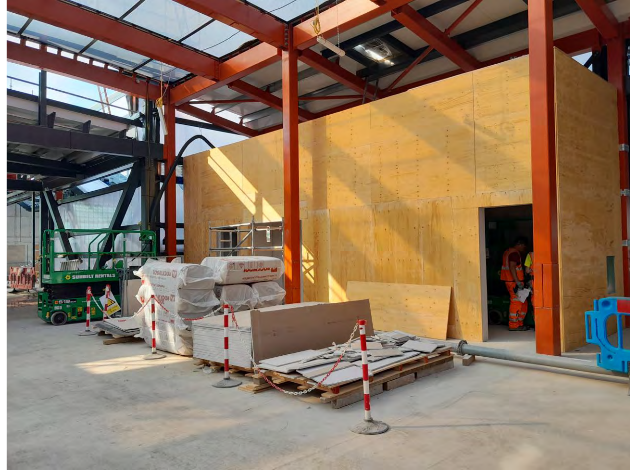
Managers room west side un-paid concourse.
