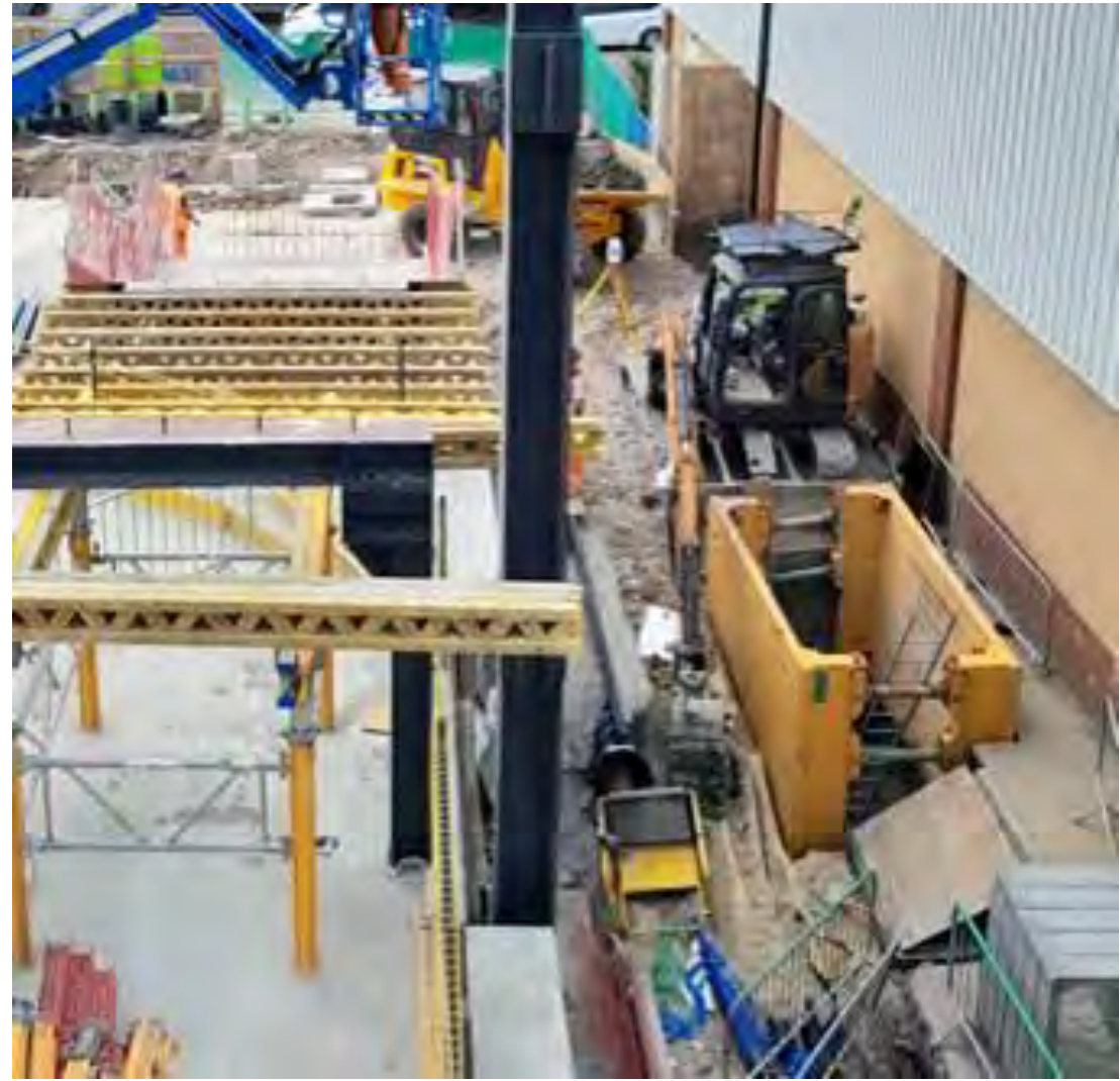
Service corridor Progression on the Western Entrance
